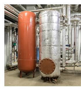
An exposed tank surface area without insulation (red colored side) results in significant heat loss.
