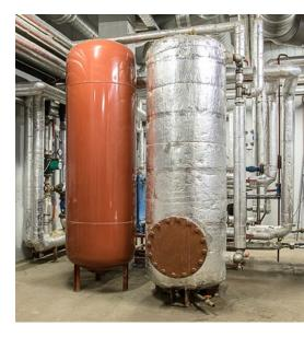
Image: An exposed tank surface area without insulation (red colored side) results in significant heat loss.
